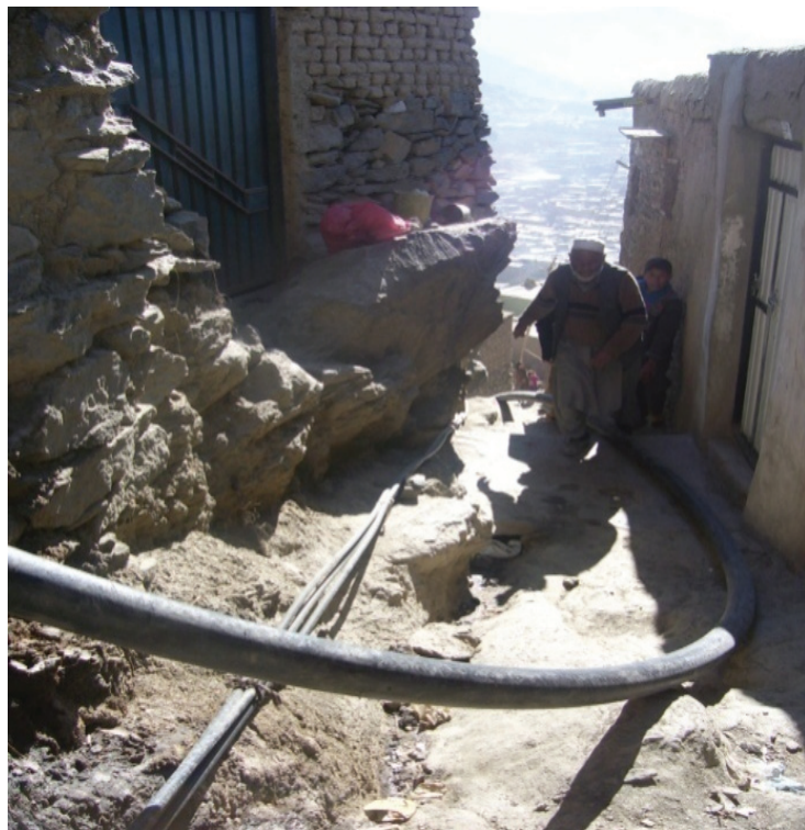
The plastic pipes, draw over ground Source: Deh Mazang, Jan 2010
